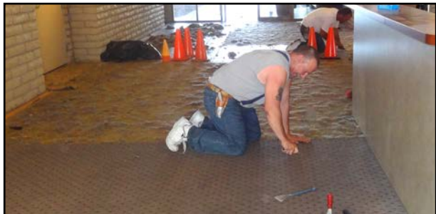
Worker installs new carpet in lobby
